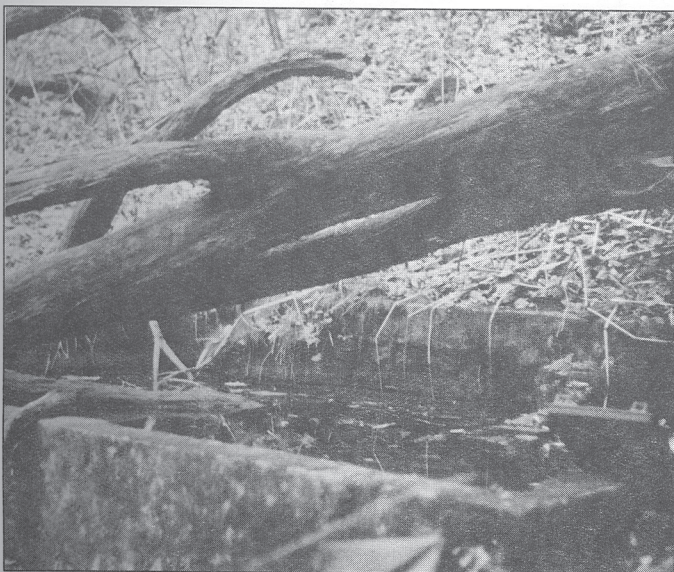
Concrete basin impounding spring #1.
