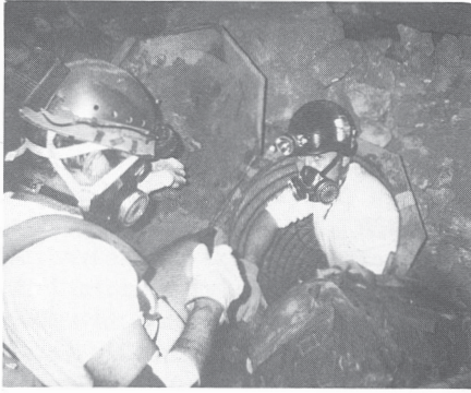
Figure 3. Andy Messer heading down the culvert wearing mask with filters.
